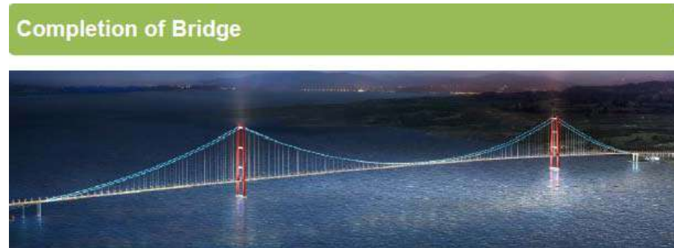
Bridge construction stages – completion of the bridge
