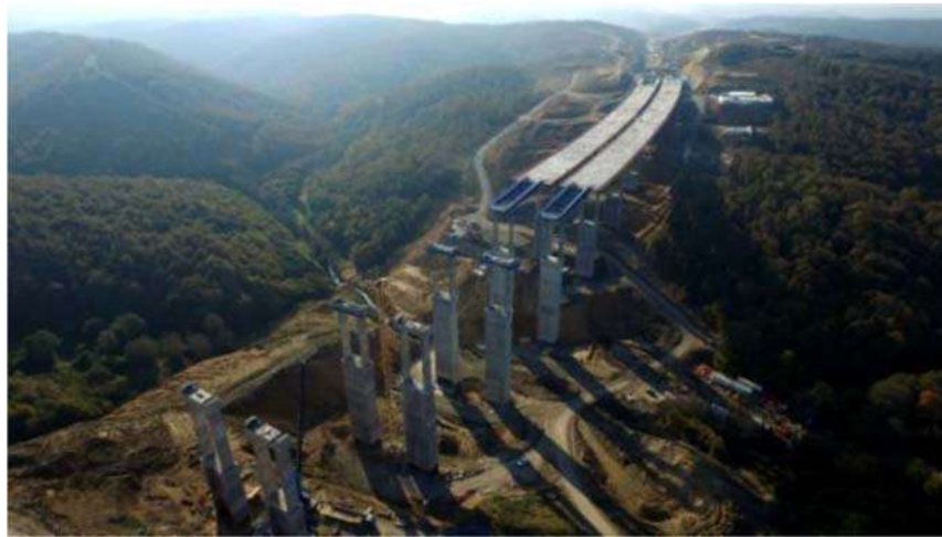
Incremental Launching Method (Illustrative Example)
