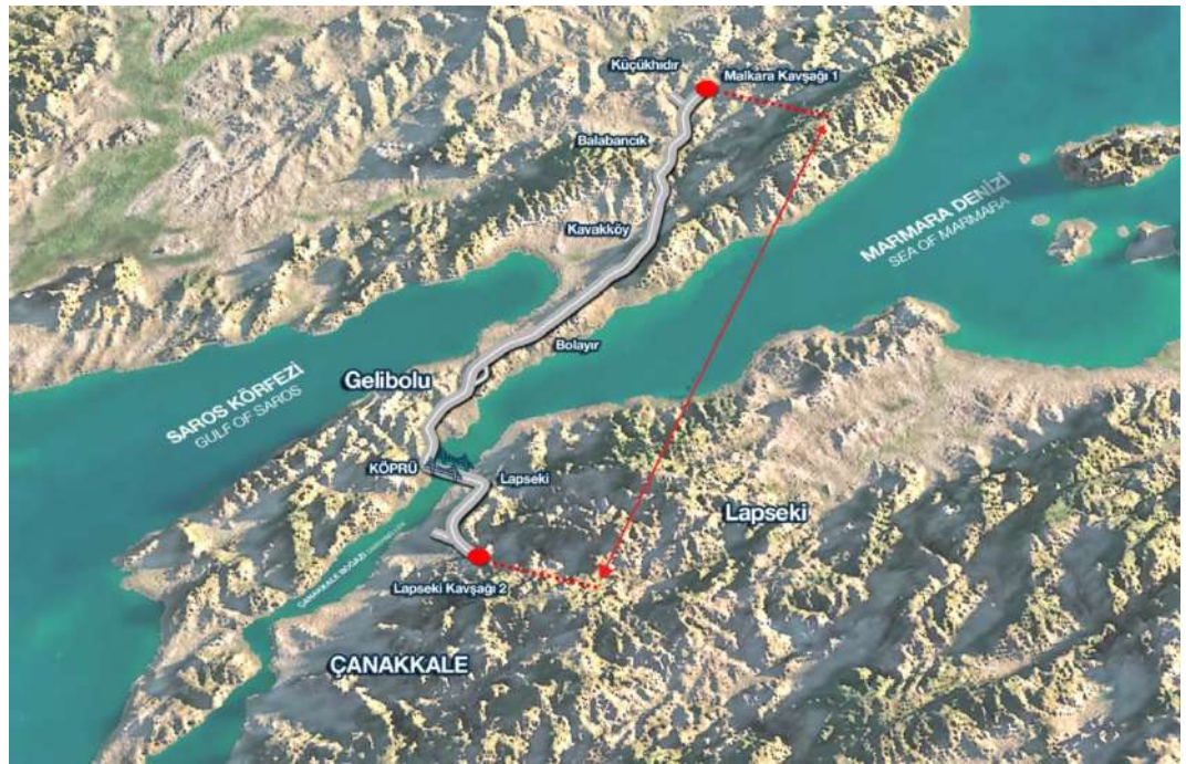
Overview of the Project (motorway section and the bridge)
